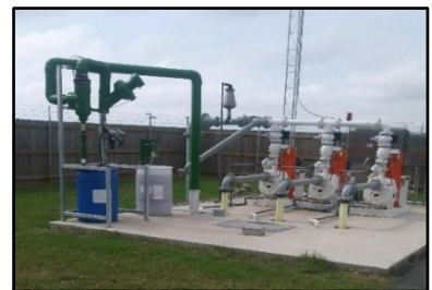
Lift Station D, located on Tower Road, lifts sewage from a low-lying area to a higher elevation so it can continue its flow to the treatment plant.
