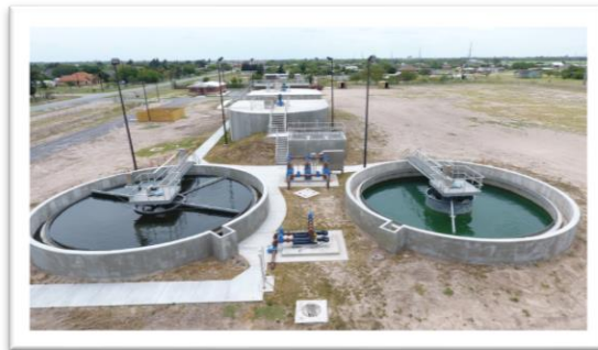
The Donna Regional Wastewater Treatment Plant became operational May 5.
